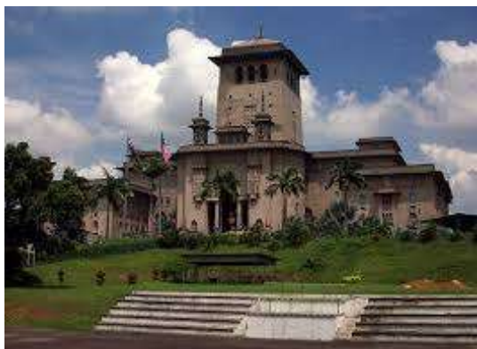
SULTAN Ibrahim Building
